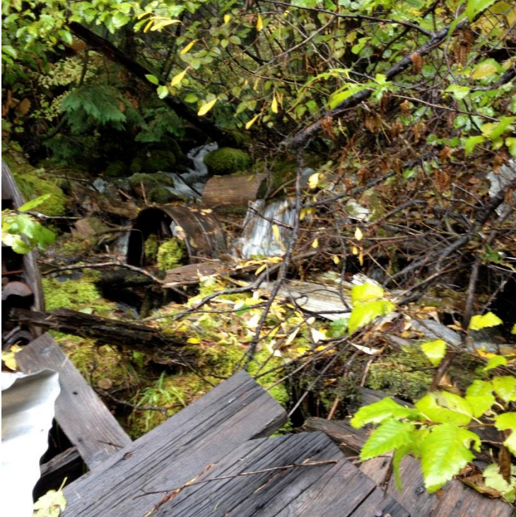
Picture 26. Unnamed tributary downstream of Bumping Dam Spillway and the passage barrier just upstream of its mouth. The infrastructure related to the old water wheel prevents passage as well as the cascade just downstream of this point (Picture 25). This barrier is considered repairable so the habitat upstream of it was included in calculations of stream habitat available to fish coming from Bumping Reservoir.
