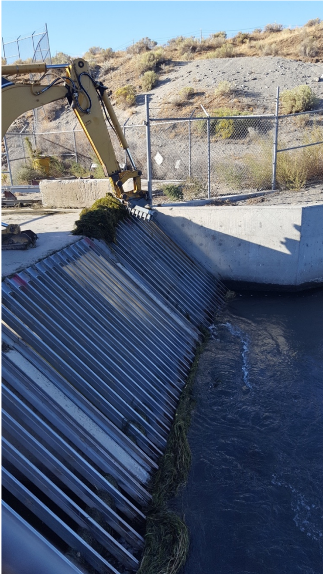
Figure 2. Photo left: Water stargrass removal at the Columbia Irrigation District Intake Screen.
