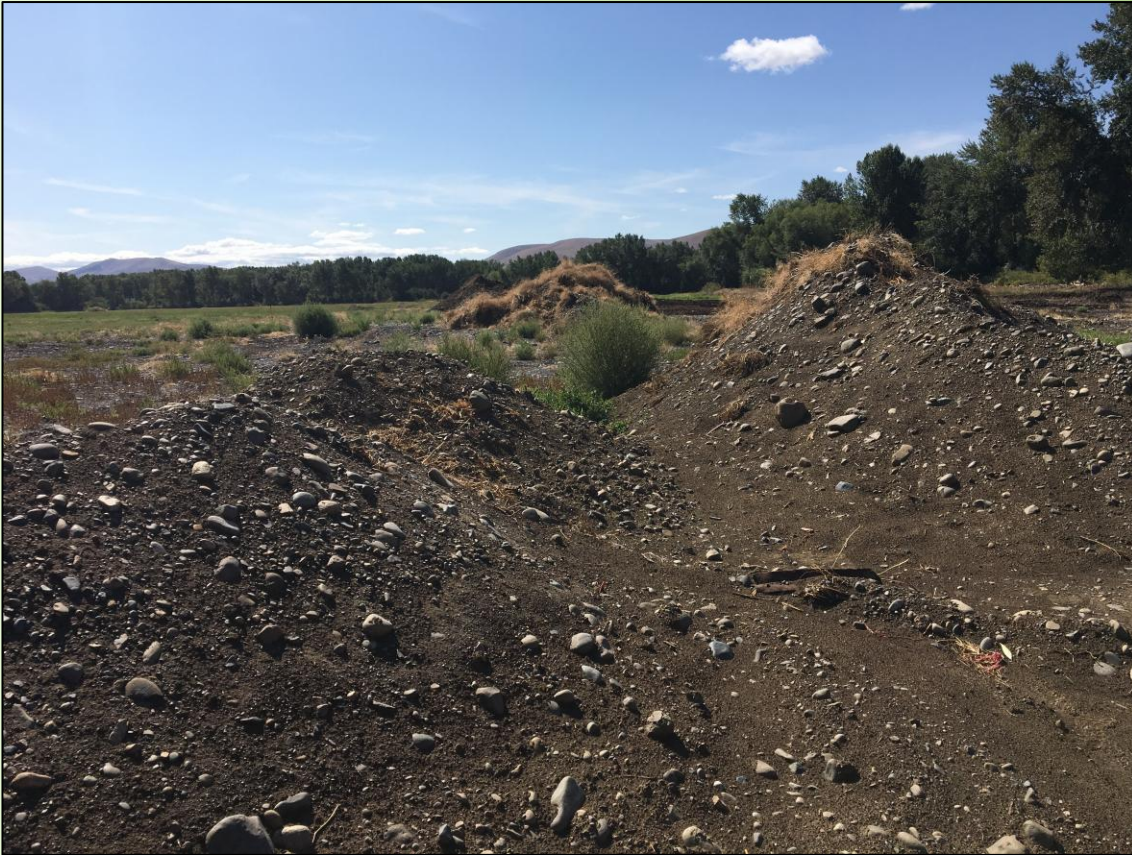
70,000 CY moved and redistributed during construction phase
