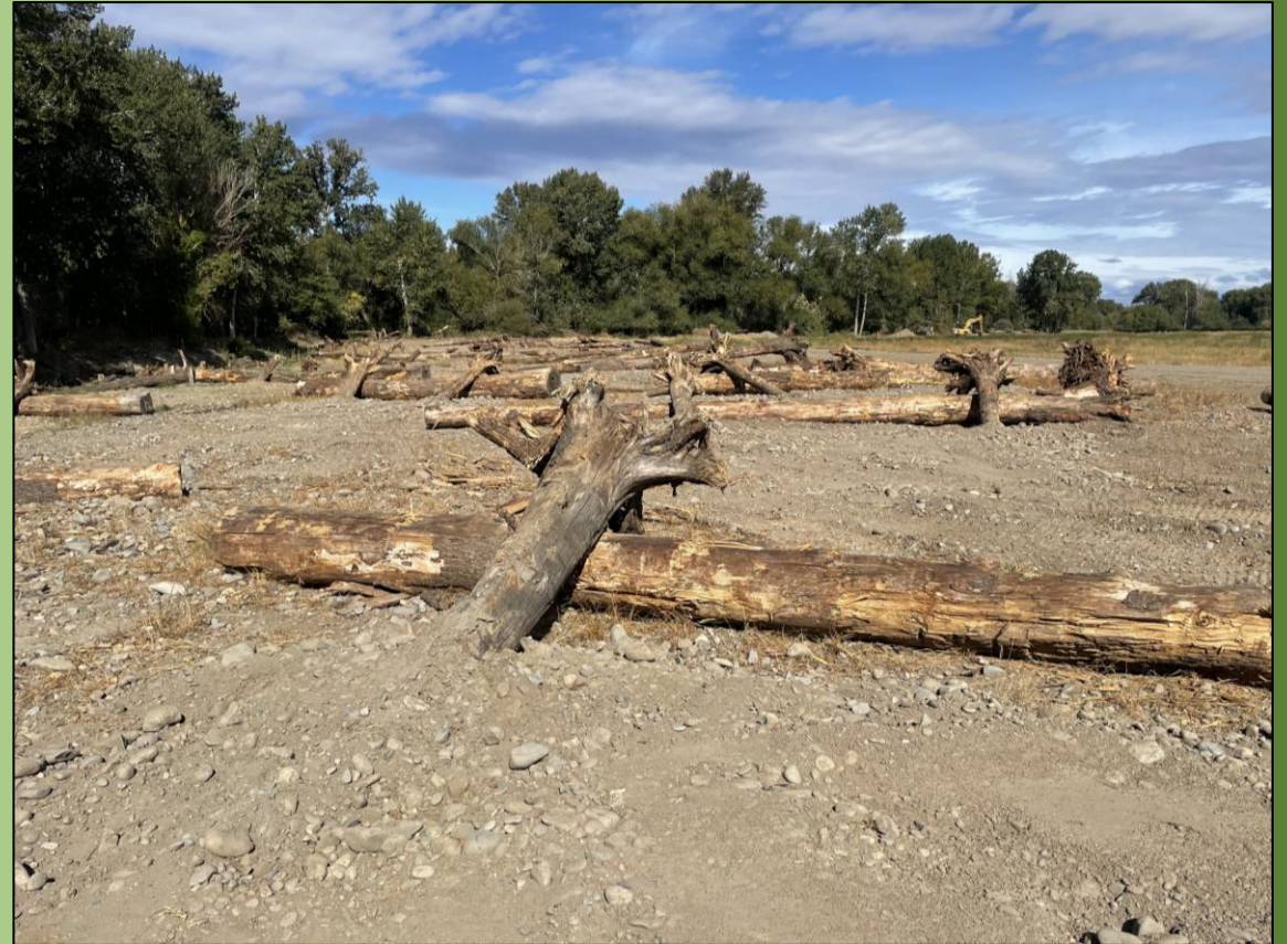
Installation of LWD after grass establishment
